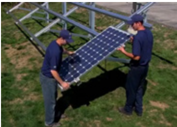
Step 6 Twist-in module clamps And secure modules
