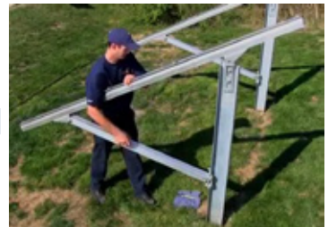
Step 4 Hang & Attach Strongback Assembly
