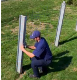
Step 2 Slide on Strut Attachment
