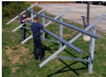
Step 5 Hand-lift module rails into place
