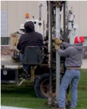
Step 1 Pile-drive I-Beams
